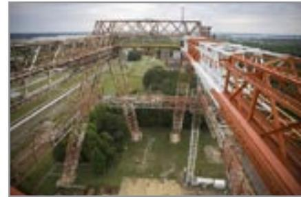
Figure 4: The gantry is receiving a fresh coat of protective paint as part of the summer renovations. Other upgrades include a new bridge, a new elevator, floor repairs and a new parallel winch system.
