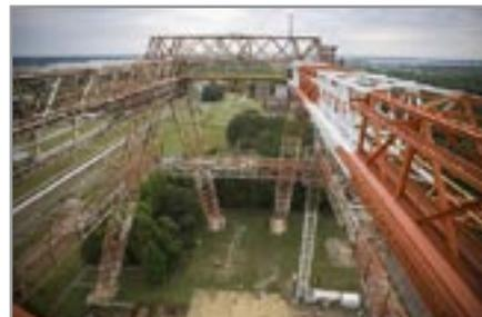
Figure 3: The gantry is receiving a fresh coat of protective paint as part of the summer renovations. Other upgrades include a new bridge, a new elevator, floor repairs and a new parallel winch system. **Image Credit:** NASA/Sean Smith
